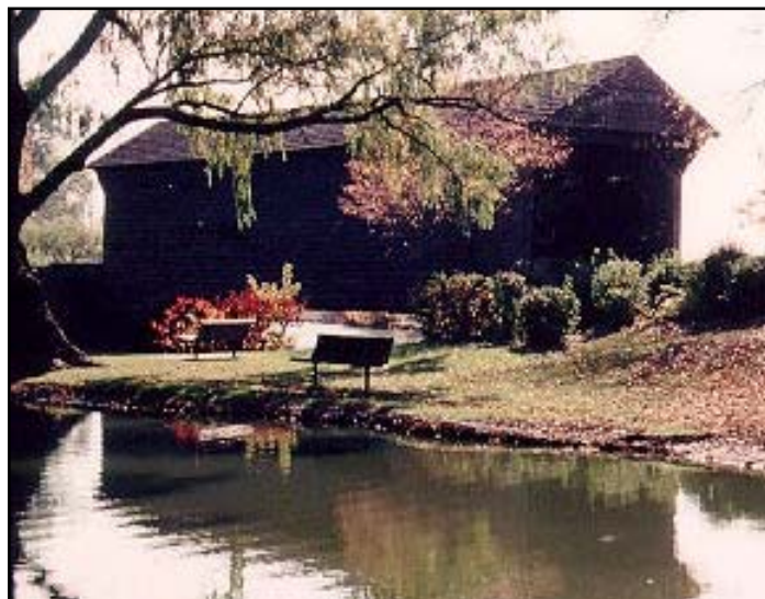
A covered bridge that Ford had moved from its original location in Pennsylvania to the Greenfield Village.
